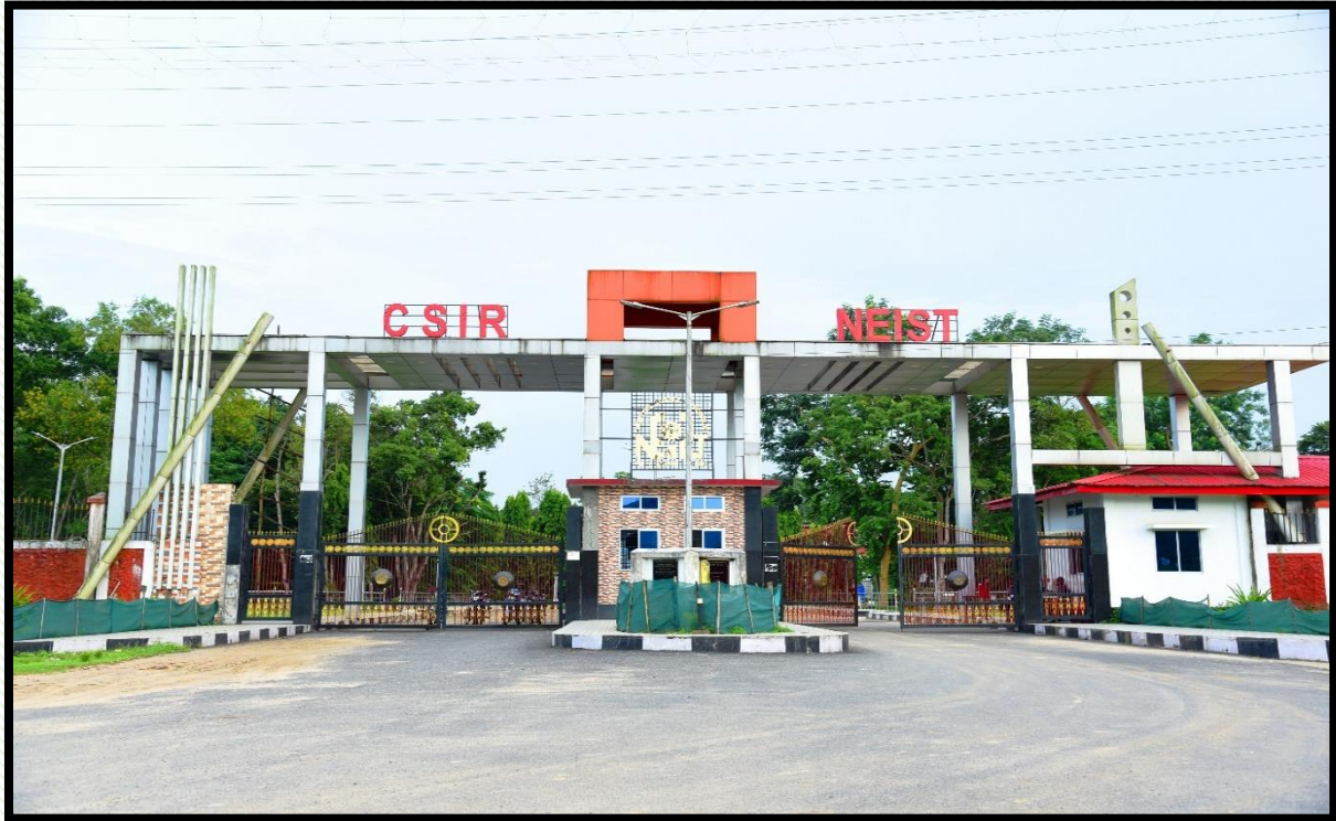
Architecturally prominent Main Entrance of CSIR-NEIST which is known as Gate No.2
